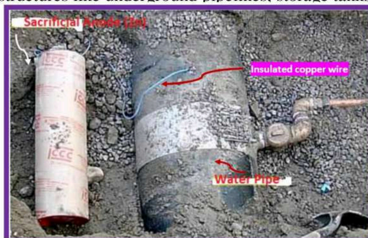
Fig. Sacrificial protection of buried water pipe.
